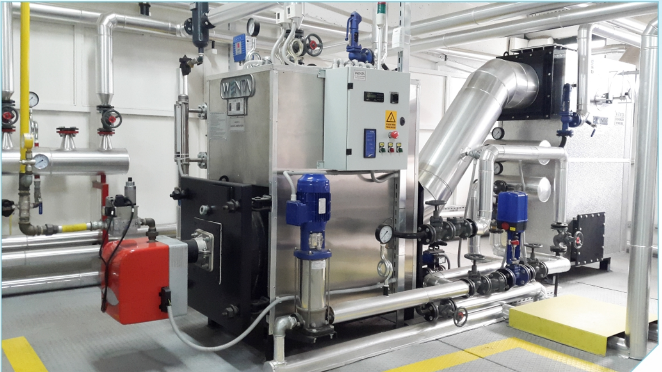
Örnek Ekonomizer uygulaması WENTA Fabrikası/ANKARA 2017. An example of Economizer application in WENTA Factory/Ankara 2017.
